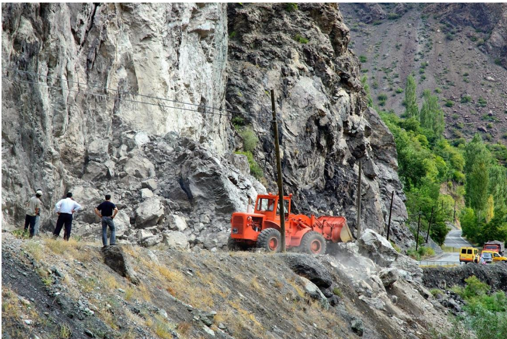
Infrastructure destroyed by rockfall after heavy rain
